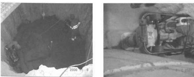
Fig.9 Emplacement of Buffer Material 'Left: Bottom, Right: Side)
