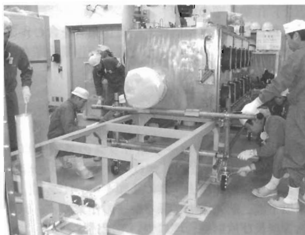
Photo 2 Separation of Gloveboxes from the Base
