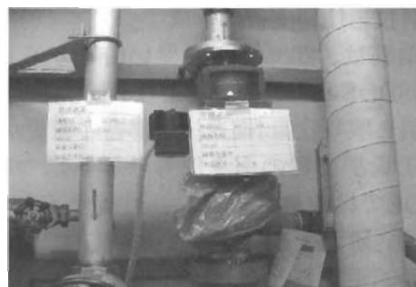
Photo 4 Isolation of Water Cooling System
