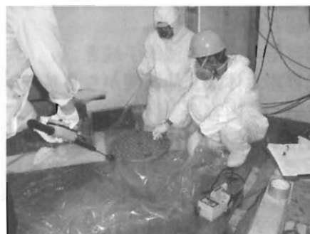
Photo 5 Radiological Survey of Installations
